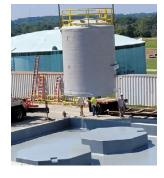
The image shows one of two bulk tanks being placed by Omega Construction. Fiberglass reinforced plastic (FRP) tanks are less flexible and hold up well to bleach, making them a better choice for the chemical. The tanks are also resistant to UV light, giving them longer life. The tanks are anchored with bolts made of Hastelloy C, a product that stands up much better to corrosion than stainless steel. This project is now completed.
